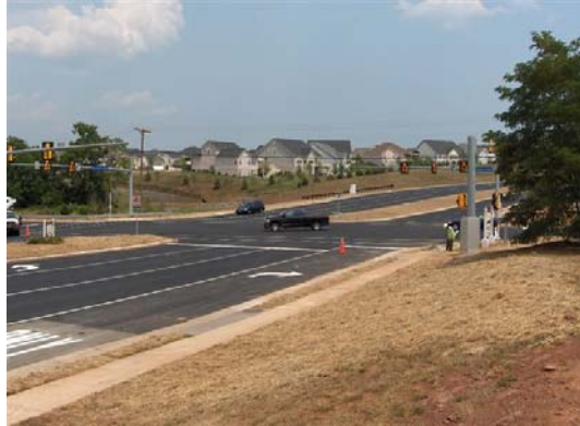
Heathcote Blvd. & Catharpin Rd. Intersection Opens 9-03-07
