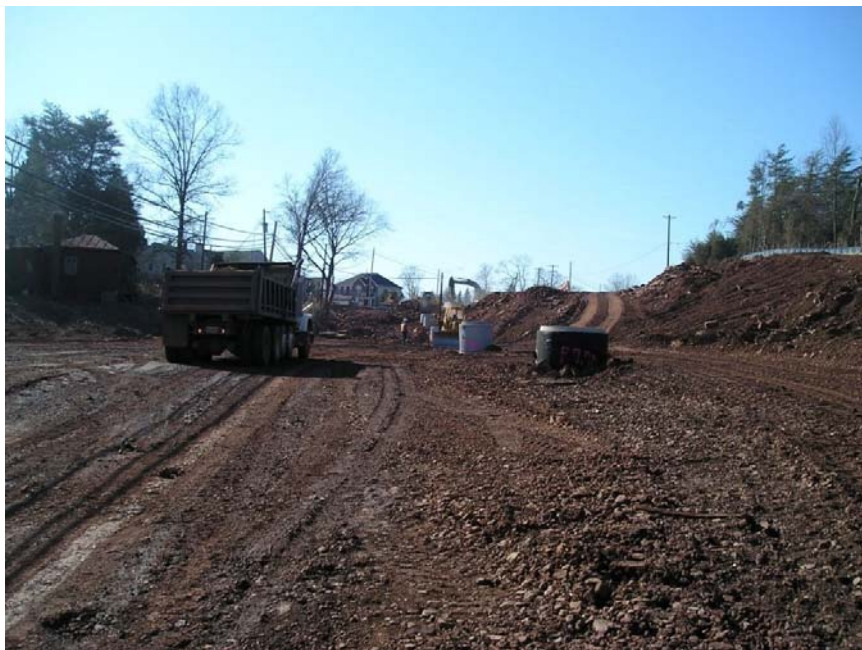
Grading work and sewer line work on Old Carolina Road
