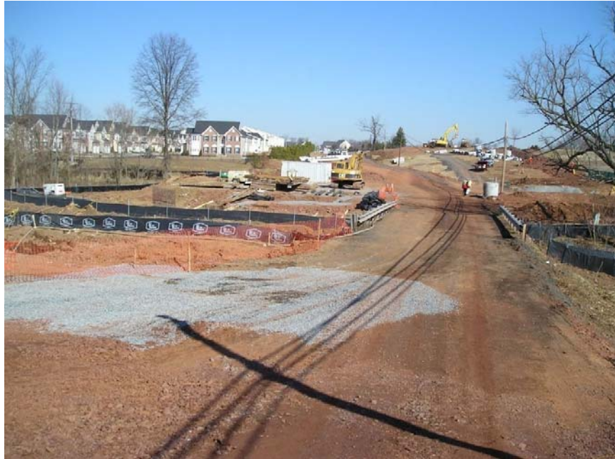
Grading work and bridge construction of Old Carolina Road
